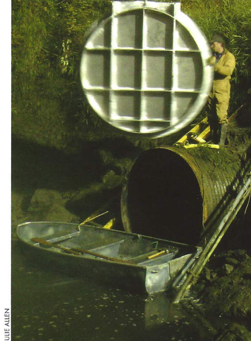
The new tide gate during installation.
