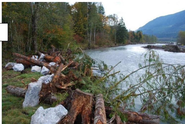
Stream bank protection work
