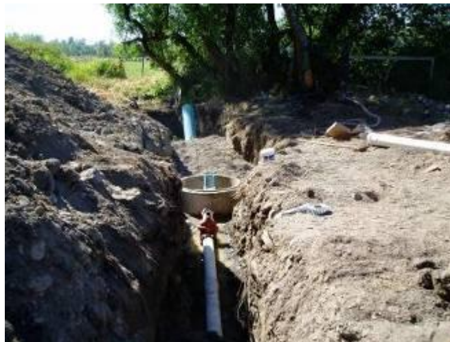
Construction underway of irrigation pipelines in Clallam County that replace older, less efficient irrigation ditches and save water in the over-appropriated Dungeness River.
