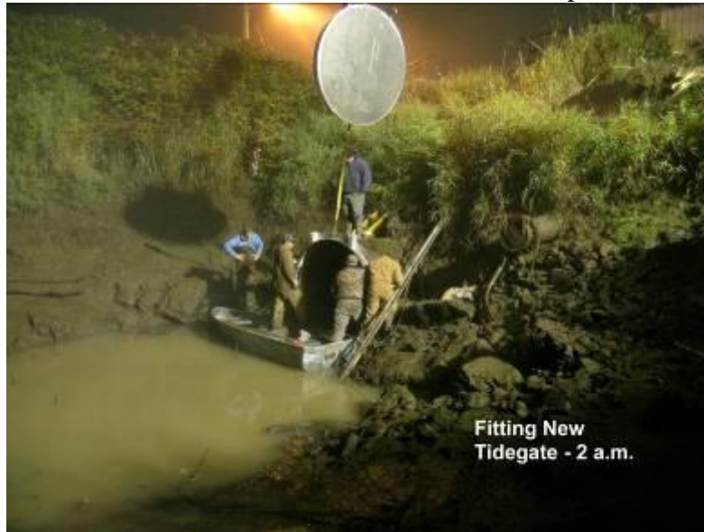
Workers installing the new, aluminum tide gate.
