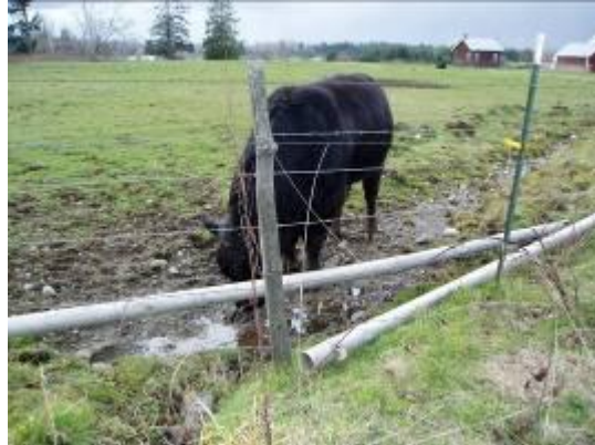
Bull in an irrigation ditch, prior to completion of the new project.
